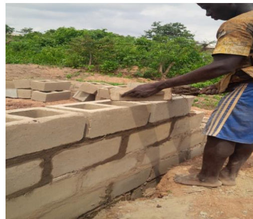
Figure 6: Mason performing laying of block
